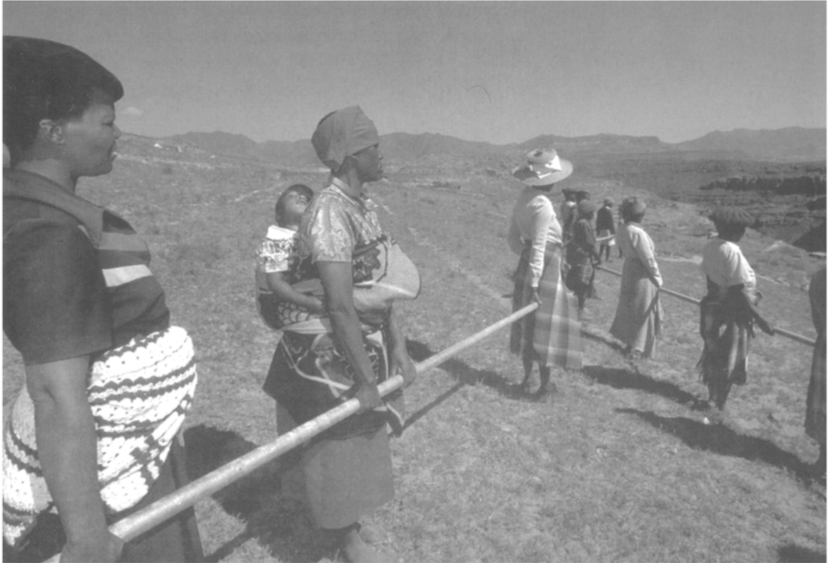
Laying water pipes in Lesotho
