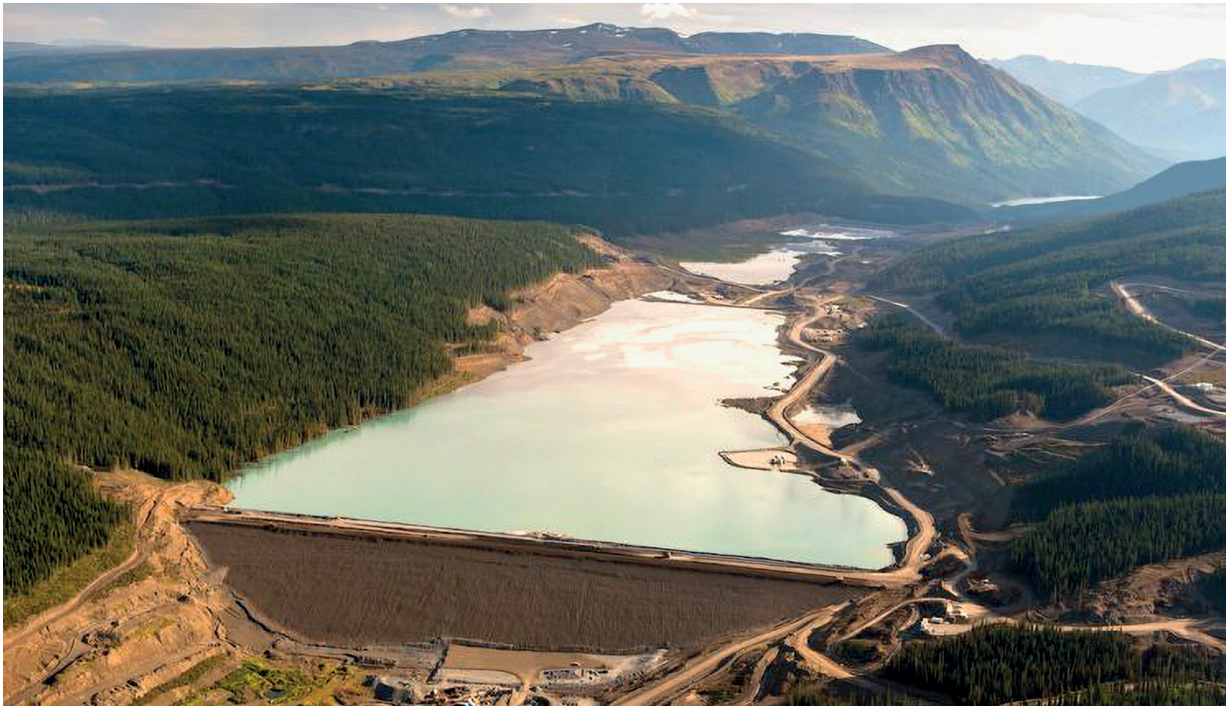
Tailings dam facility in British Columbia, Canada [photo credit: Garth Lenz]
