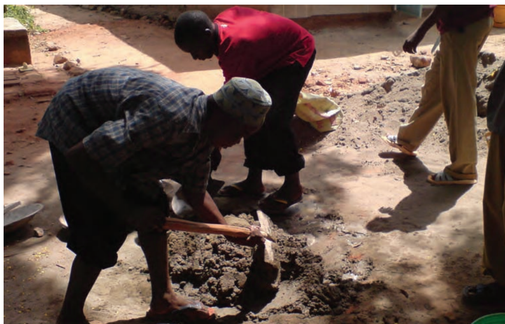
Building new classrooms in Kisarawe, Tanzania.
