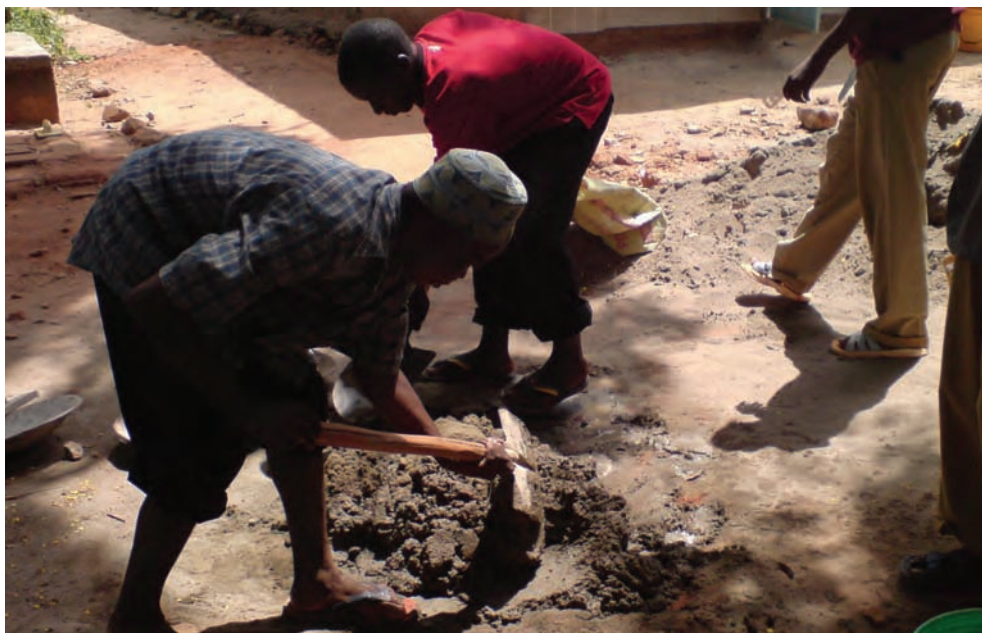
Building new classrooms in Kisarawe, Tanzania.
